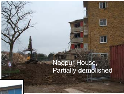
Site Hoarding erected along Bell Road
